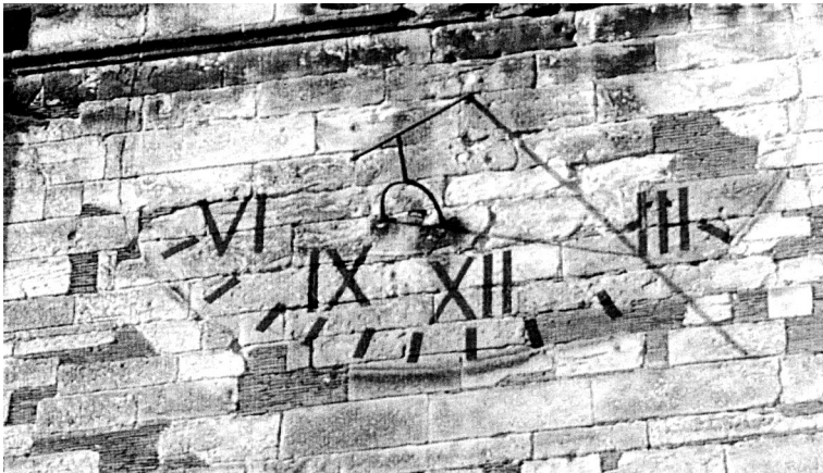
Photo 2: after completion of the restoration
